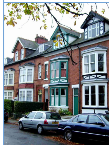
Daneshill Road, Western Park
